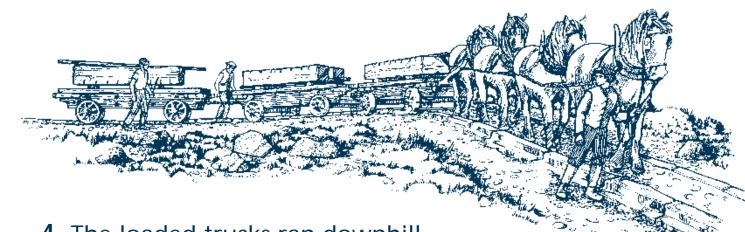
4 The loaded trucks ran downhill from Haytor to Ventiford on the Stover Canal, but they had to be brought uphill from Holwell Quarry. Teams of horses were used to pull trains the short distance up from Holwell to the point where gravity could take over. The trucks had no brakes but braking was carried out by levering long poles against the wheels.
