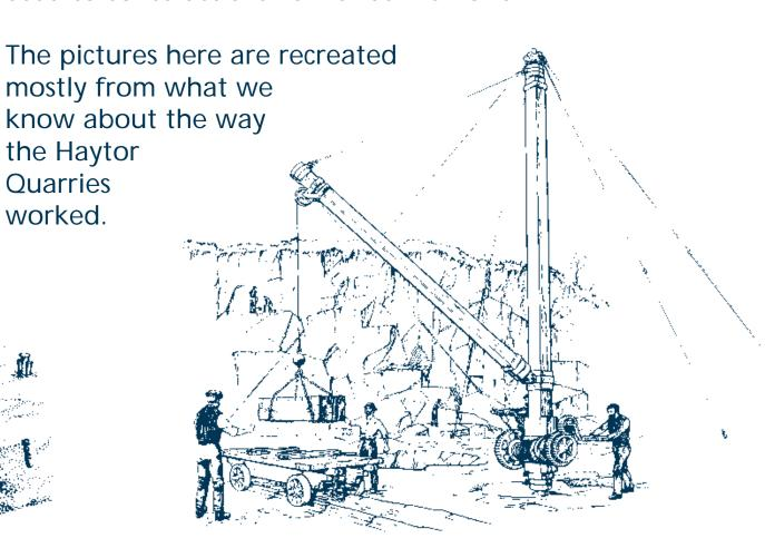
3 The large blocks of granite were lifted onto flat-topped trucks by means of a derrick (remains of the derrick illustrated can be seen at Haytor Quarry). This was operated by hand and had two gear trains. The whole unit pivoted on a metal bearing sunk into the granite (still visible), the top being held vertical by metal rods which were joined to allow flexing under the load.
