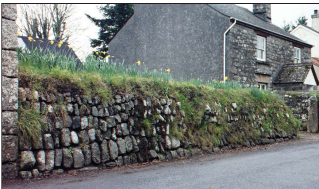
Figure 24 Stone-faced bank adjacent to Castle House
