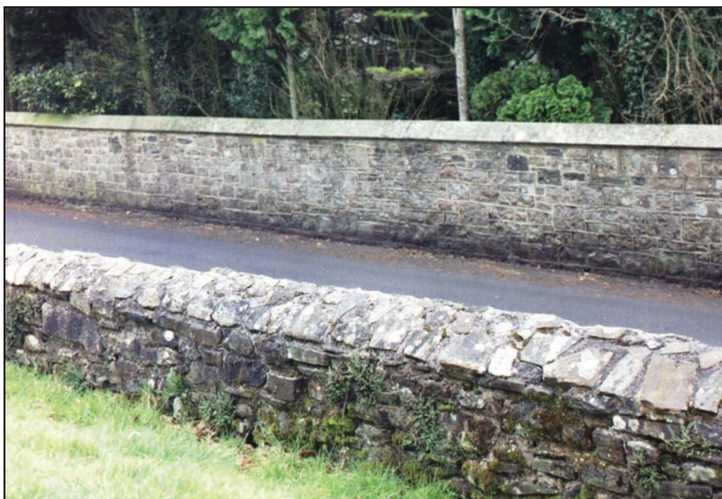
Figure 22 The wall of the castle (foreground) and former vicarage
