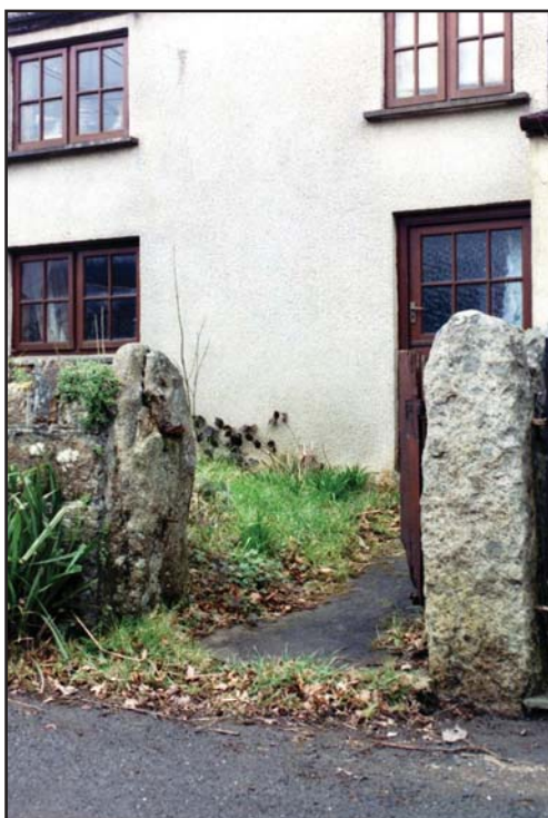
Figure 23 Gate posts at 1 Rose Cottage
