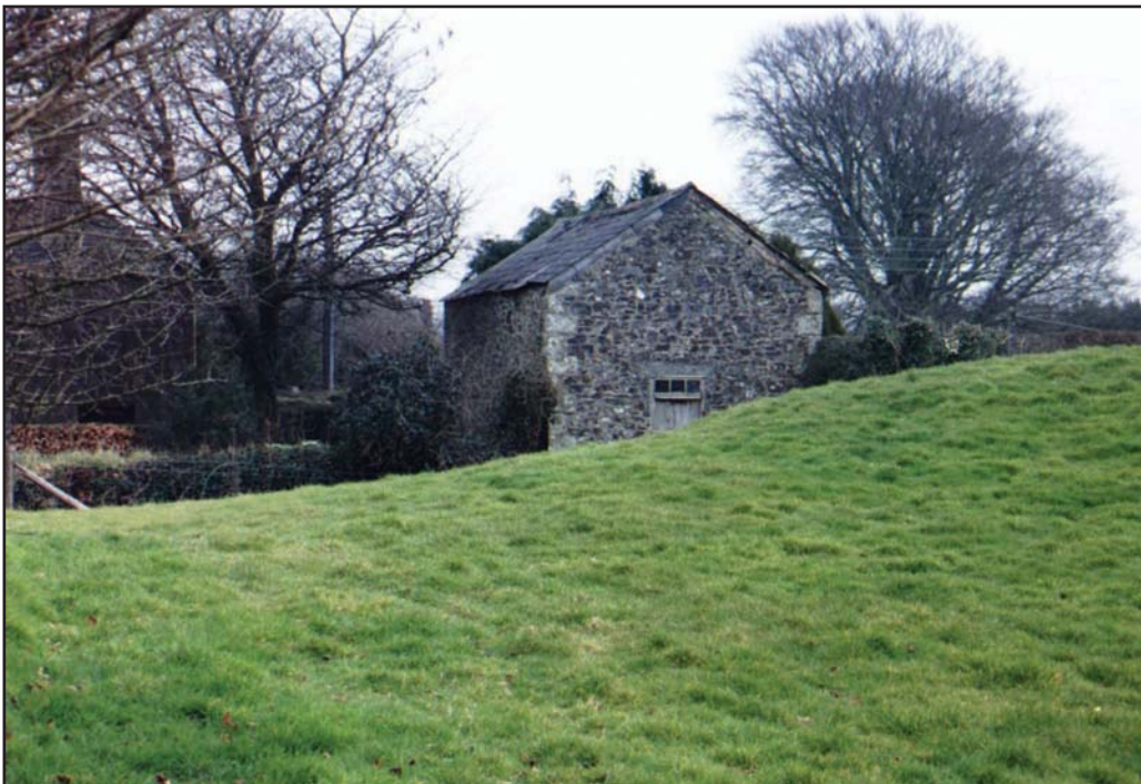
Figure 2 Small outbuilding S of main street behind Lydonia
