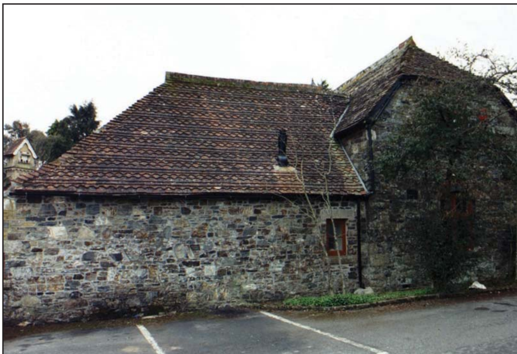
Figure 6 The former Vicarage stable block
