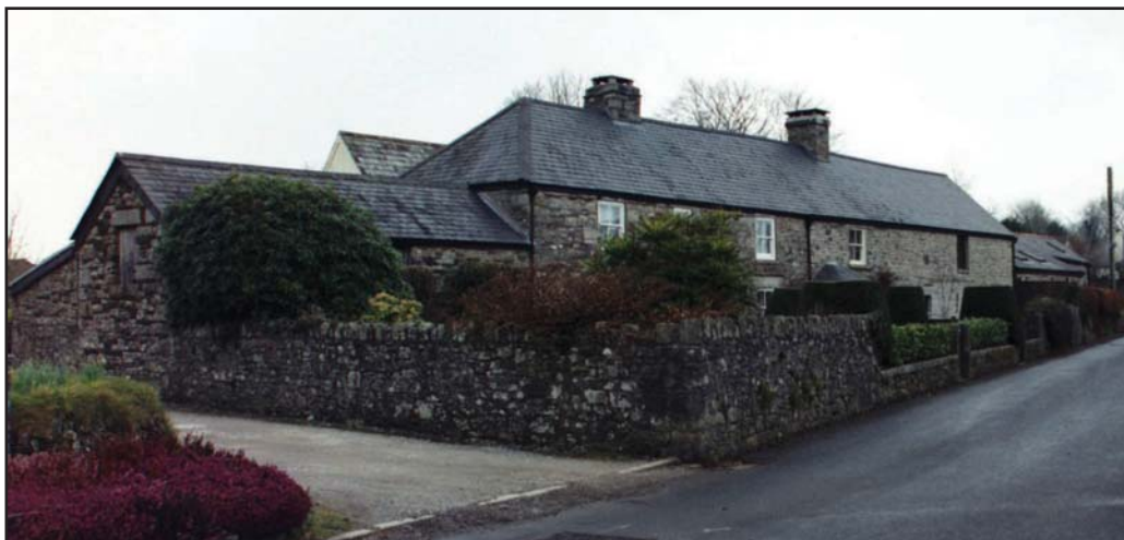
Figure 15 The range of buildings at Town Farm
