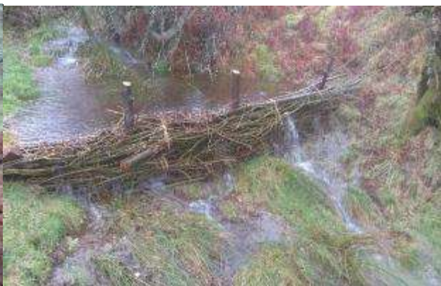
Trial leaky dams installed winter 2019/2020
