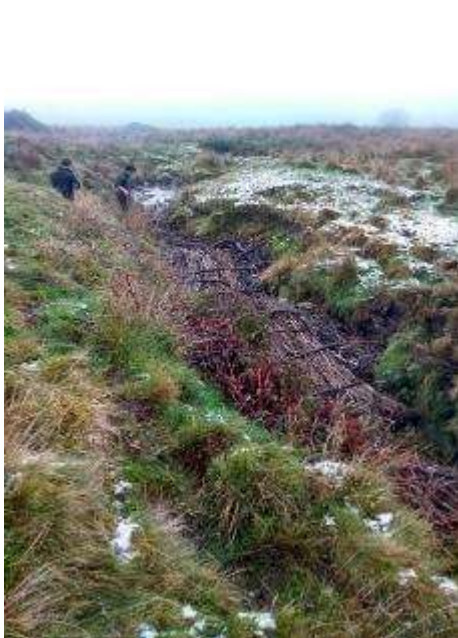
Willow faggots used to slow the flow
