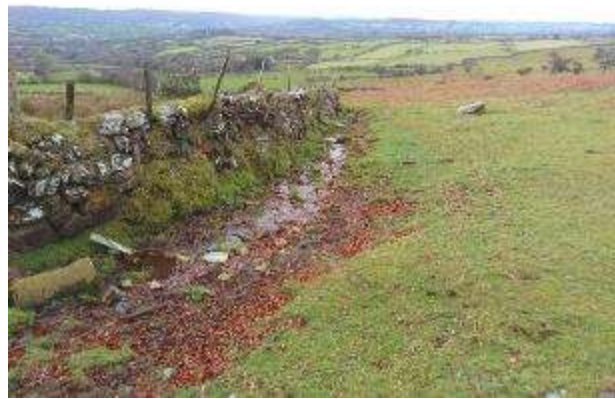
Water channelled by the stone corn ditch
