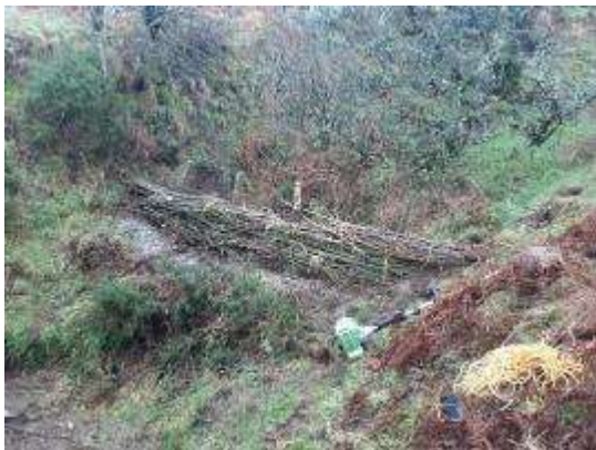
Trial leaky dams installed winter 2019/2020
