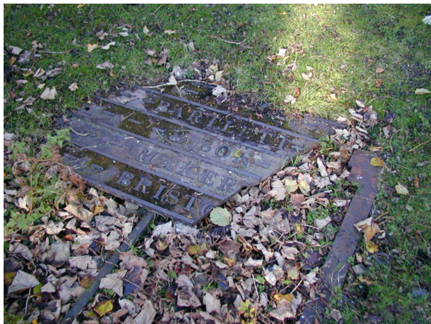
The remains of the base plate of the weigh-house (Photo: Kevin Page 2005)
