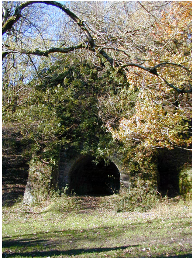
The larger western limekiln (Photo: Kevin Page 2005)
