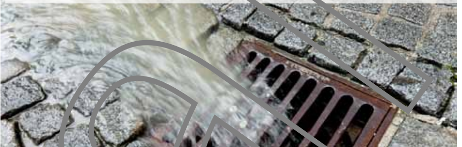
2 - DRAINAGE GRATING CONNECTING OVERLAND FLOW TO CULVERT
