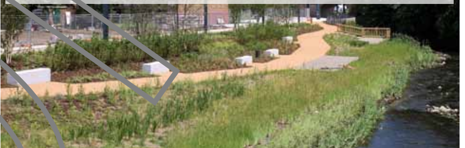
4 - RIVER BANK REPROFILED TO INCREASE CONVEYANCE
