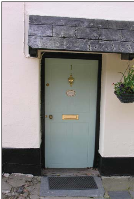
Figure 9 Flush panelled door.
