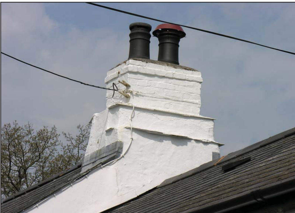
Figure 6 Stone stack with brick top.
