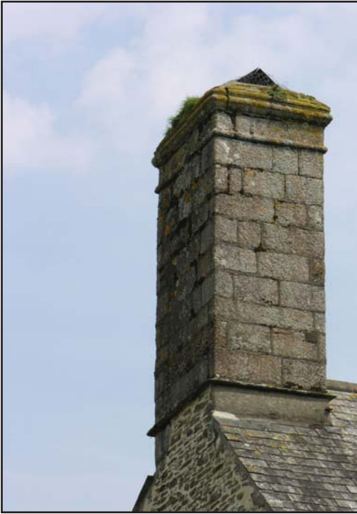
Figure 5 Dressed granite chimney at the Barton.
