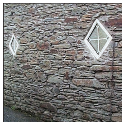
Figure 19 Loss of detail: inappropriate PVCu windows
