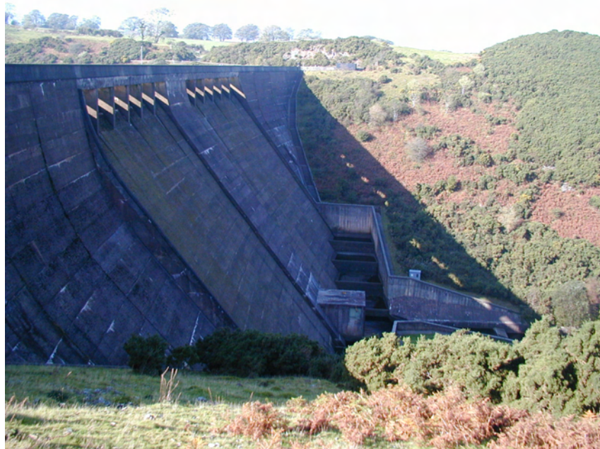
Meldon Dam from the south-east (Photo: Kevin Page 2005)
