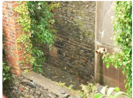
S wall, C2, showing earlier masonry at base
