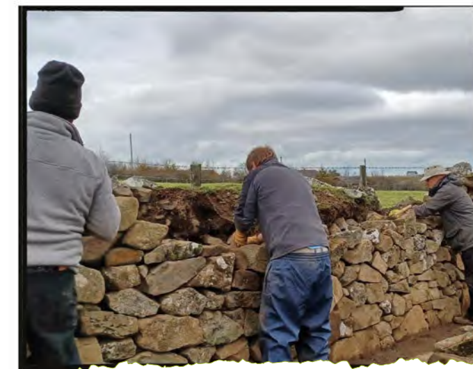
Drystone walling, Okehampton Common, Dartmoor Hill Farm Project
