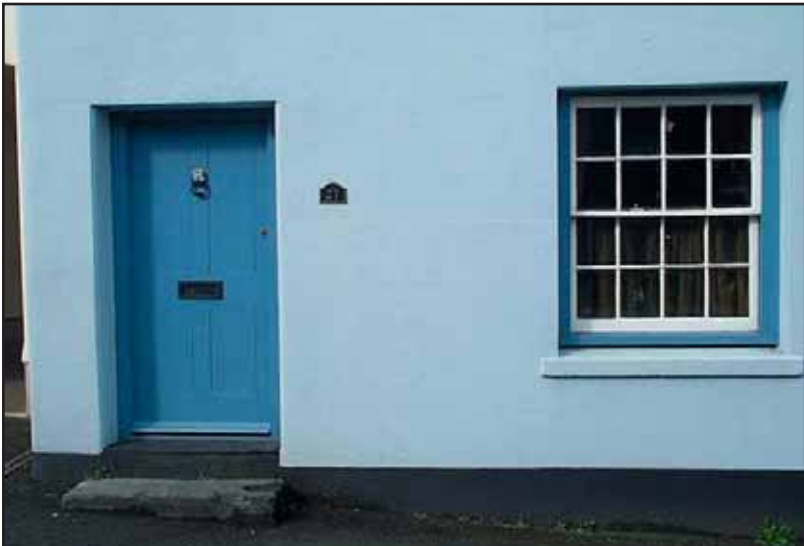
Fig 15 Georgian sash window and panelled door
