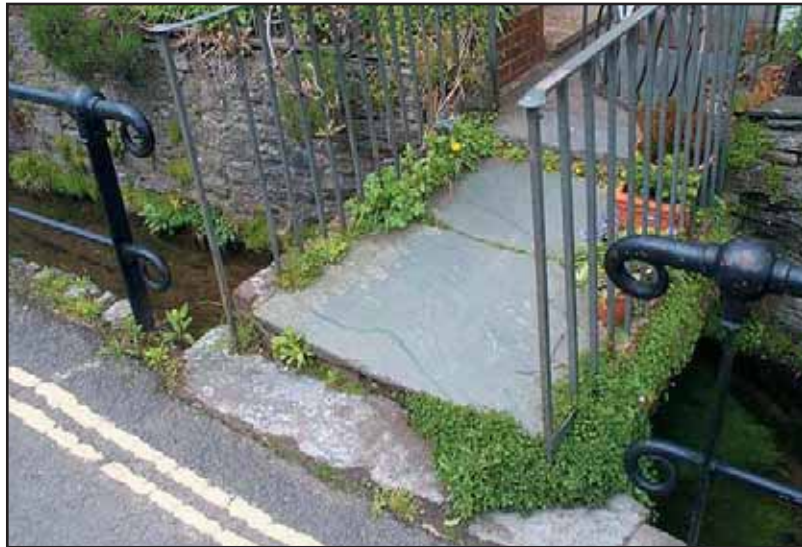
Fig 60 Slate slab bridge over the Town Mill Leat
