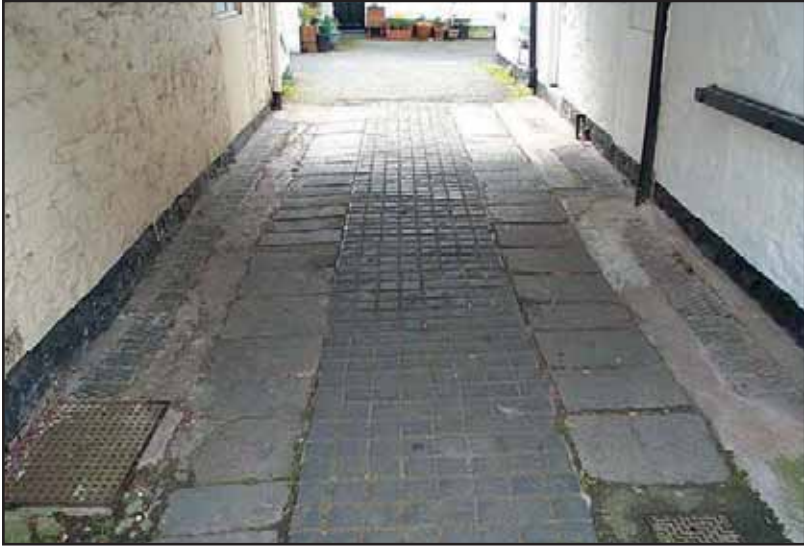
Fig 56 Granite slabs and blue pavements in an ope
