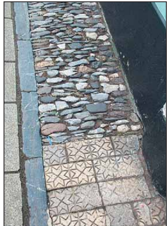
Fig 55 Cobbles and buff paviours on Fore Street
