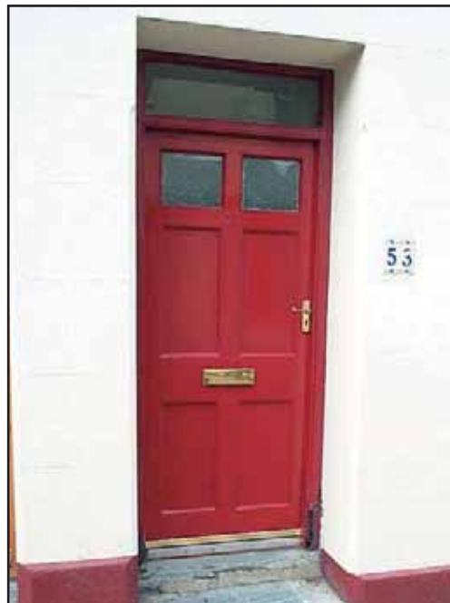
Fig 17 Victorian panelled door with limestone step
