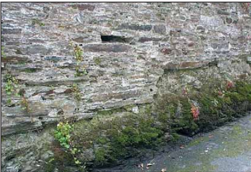
Fig 62 Rubble stone wall built on slate bedrock at Crest Hill
