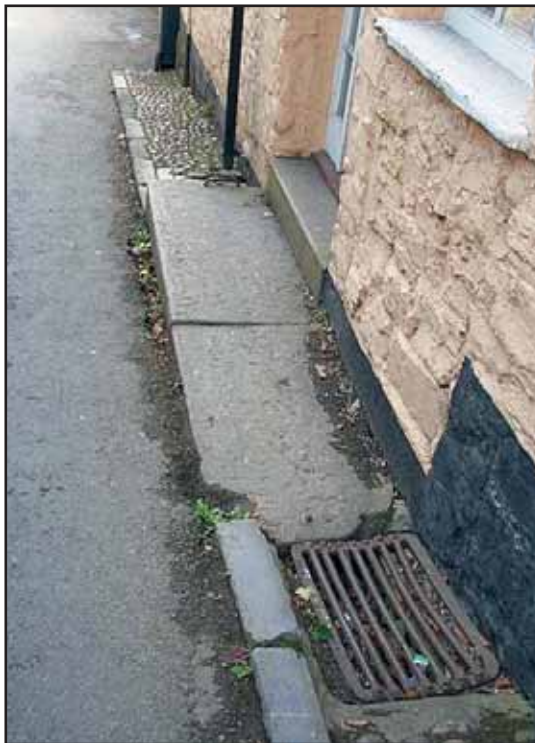
Fig 54 Cobbles, granite steps and limestone kerbs at Silver Street
