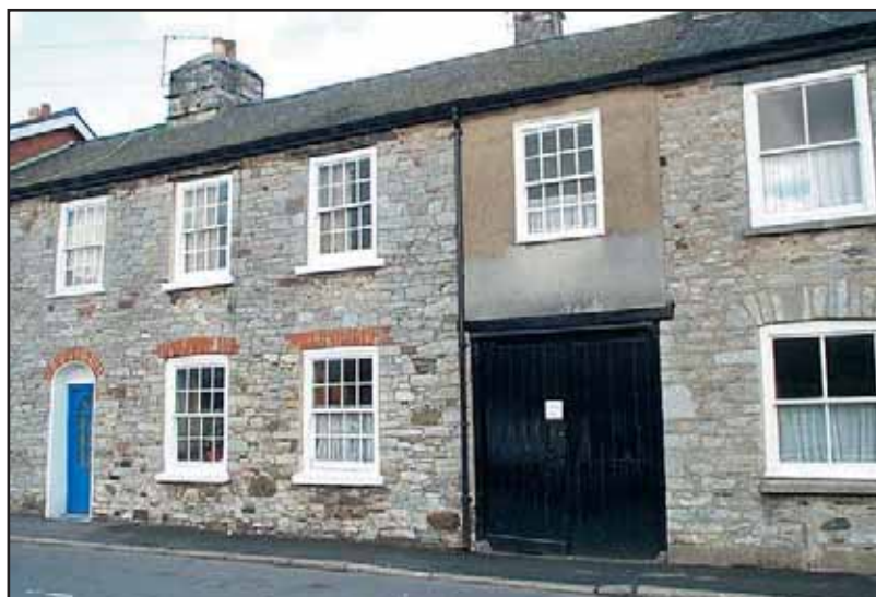
Fig 10 Typical limestone construction, formerly rendered
