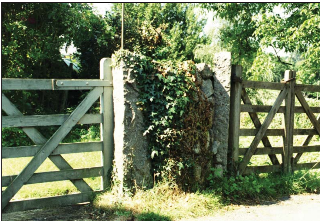
Figure 20 One each of two pairs of granite gateposts near Lower Wreyland
