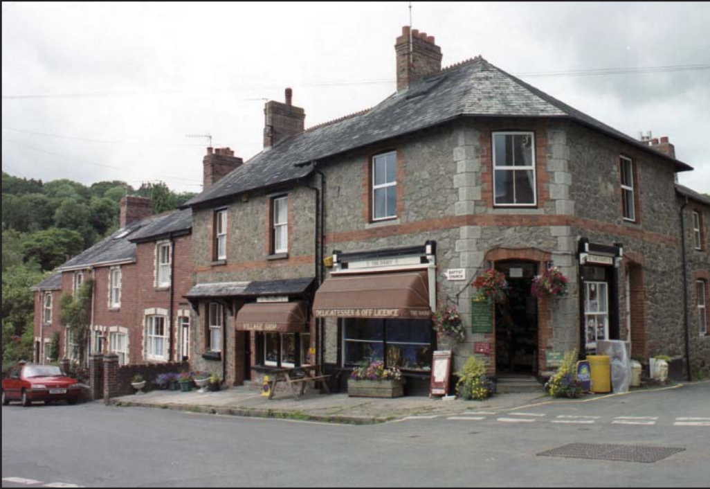
Figure 17 The Dairy and next door cottage
