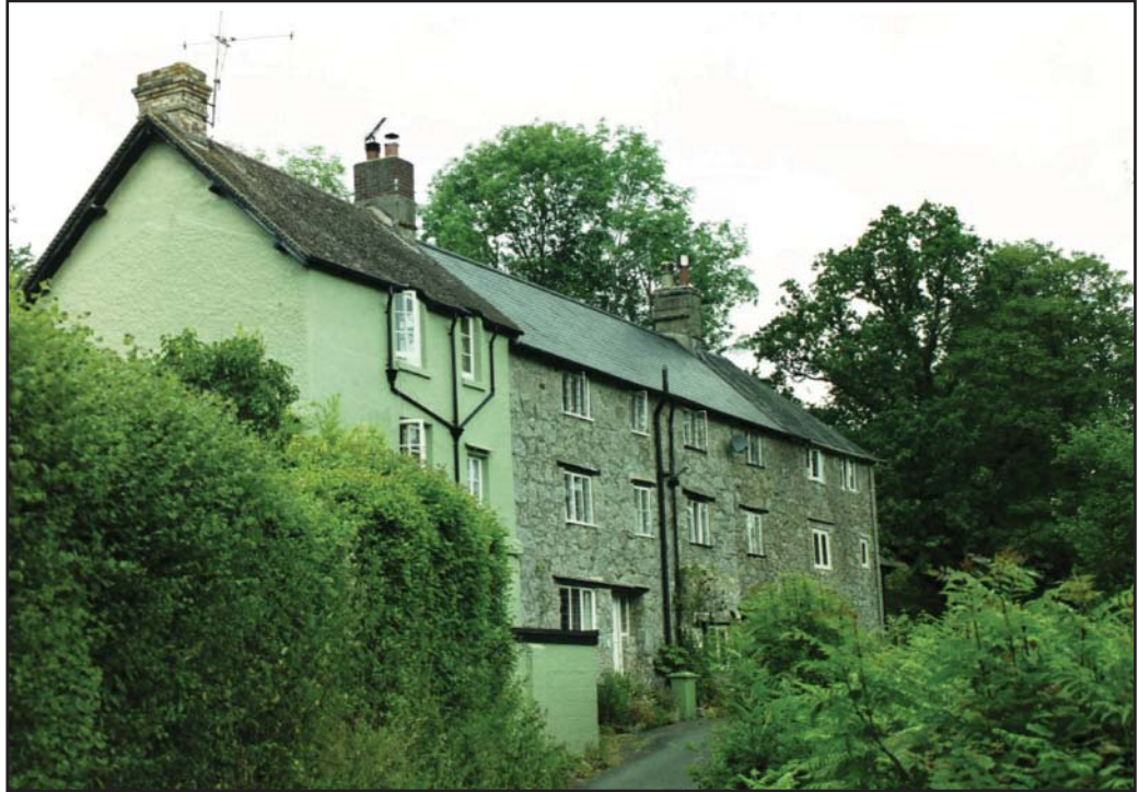
Figure 13 1, 2 and 3 Rock Cottages
