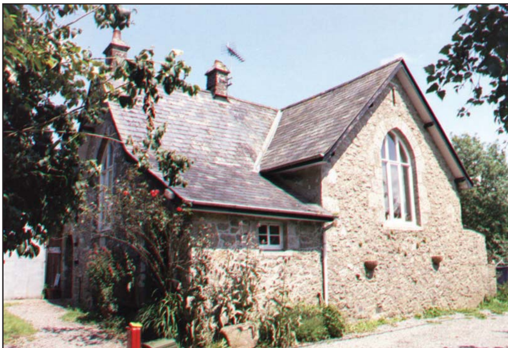
Figure 13 Church House School
