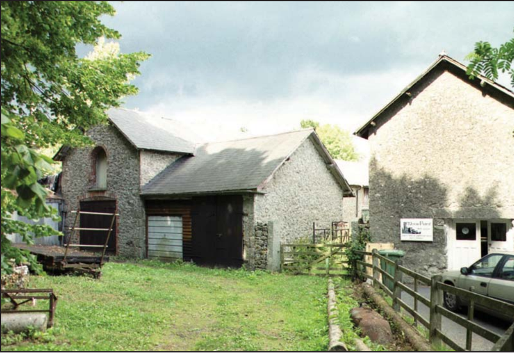
Figure 16 Town Barton farmbuildings
