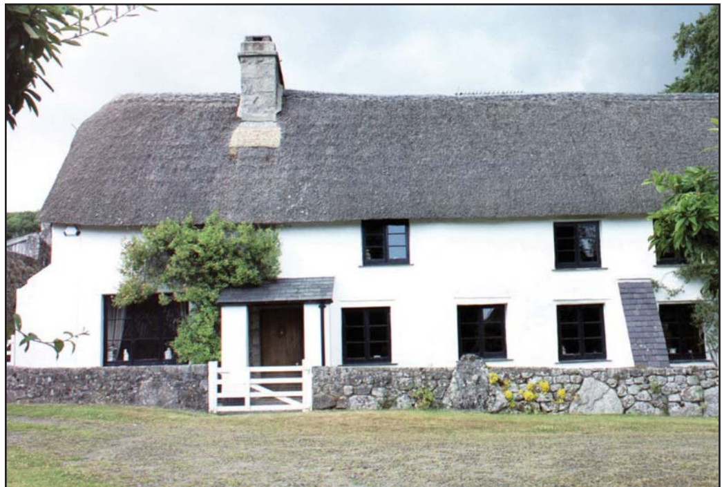
Figures 2 and 3. The long, low proportions, flush casement windows and thatched roofs of Church Cottage (top) and Half Moon (above) are typical of their medieval age, but one has its granite walling exposed and the other has it clad in (painted) render.
