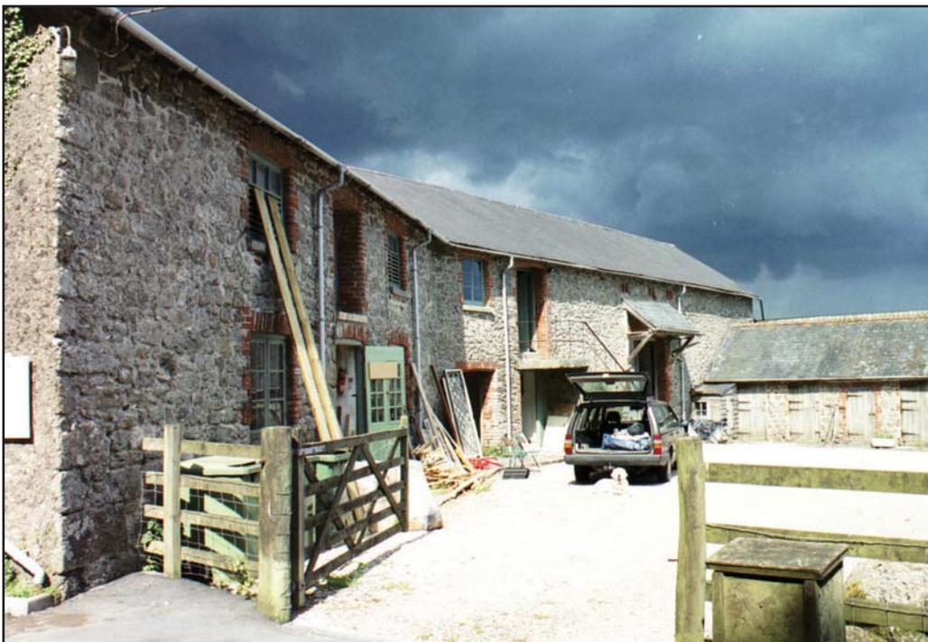
Figure 4 Town Barton farmbuildings
