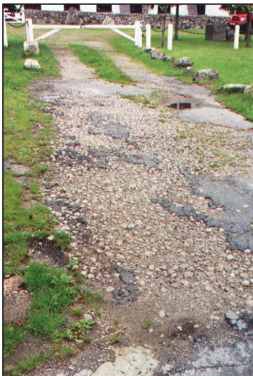
Figure 27 Exposed area of cobbles
