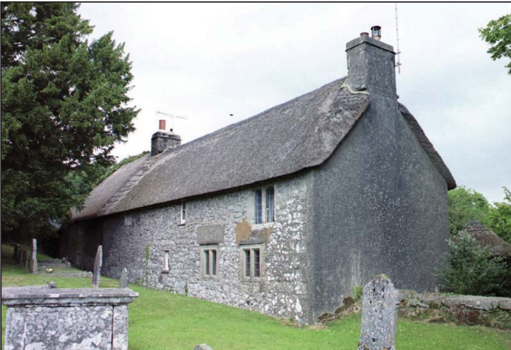
Figure 10 Rear elevation of Church Cottage
