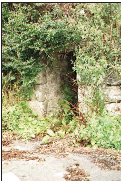
Figure 17 The Well built of granite
