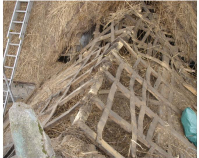
An historic roof uncovered as part of an investigation into its origins and condition. Recording of the structural arrangement and condition will be made before any conservation or renewal work is carried out whether as repairs or as approved changes to the structure. © DNPA
