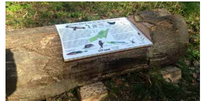
Interpretation panel set in reclaimed storm damaged timber. 3mm enviro panel bonded to 18mm marine ply panel.
