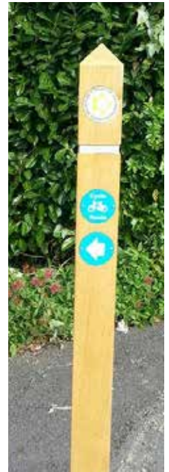
Above example of an oak way marker with inset acrylic discs identifying direction and cycle route.
