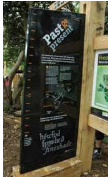
Above detail of aged steel interpretive panel and enviro panel mounted in oak support frame.
