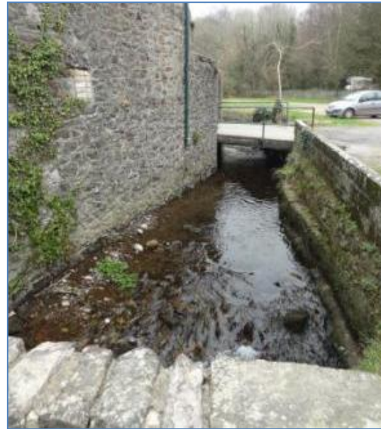
Figure 3 – River Ashburn in south of Chuley Road site
