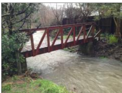
Figure 35 –Small privately owned footbridges at south of Stonepark Crescent
