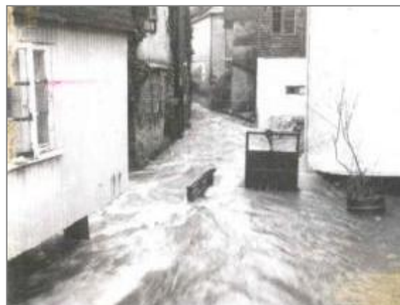
Figure 11 – Flooding in centre of Ashburton at Kings Bridge. 11.2.1974.
