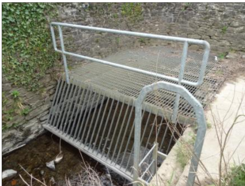
Figure 4 – Inlet to Balland Stream culvert
