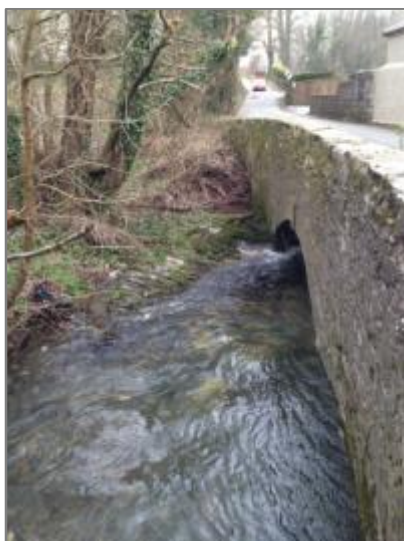
Figure 33 – Old Totnes Road bridge
