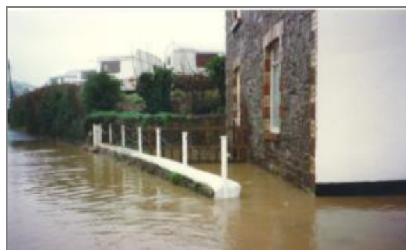
Figure 9 – Flooding in Chuley Road to south of Caravan Park, 7.2.1990
