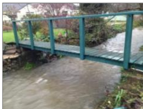
Figure 36 –Small privately owned footbridges at south of Stonepark Crescent
