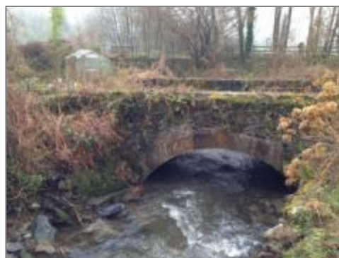
Figure 34 - Small arch bridge 20m upstream of Castle Bridge
