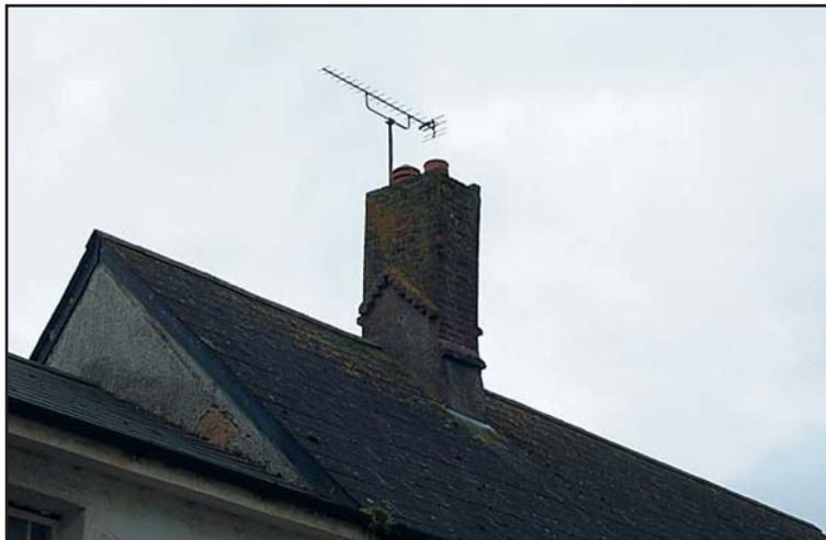
Fig 5 Chimney with brick drip course showing the height of the former thatched roof at The Old Post Office
