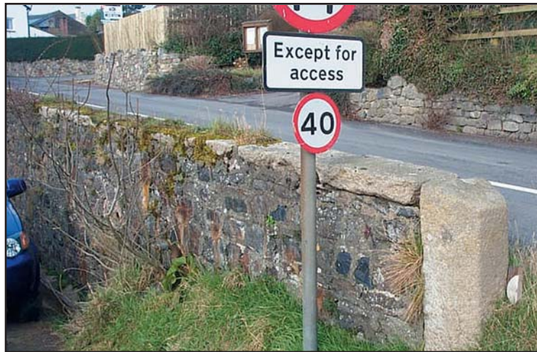
Fig 17 Retaining wall with granite post
