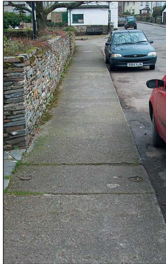
Fig 27 – Concrete slabs cover the leat.
