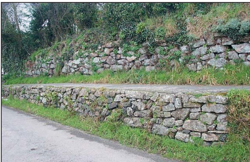
Fig 28 – Raised pavement on Tawton Lane.
