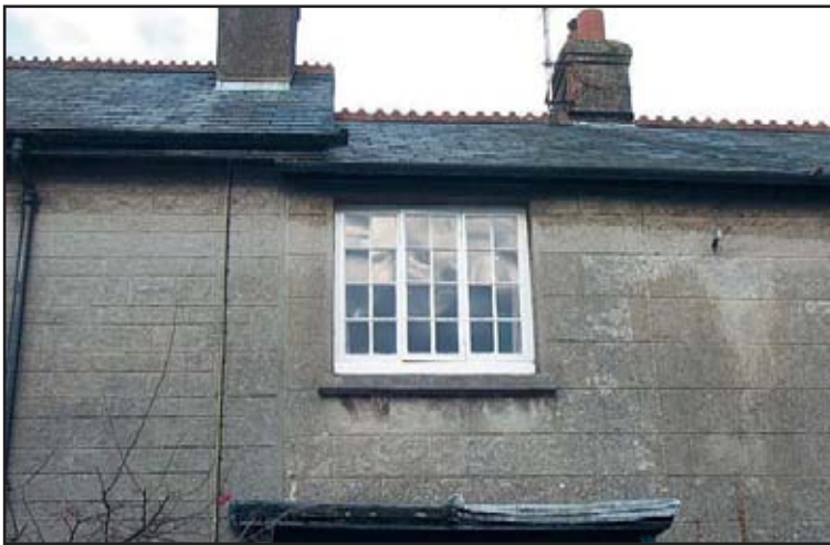
Fig 10 – The ridge, eaves, windows and canopy of Park House and Cottage epitomise 19th century re-modelling.
