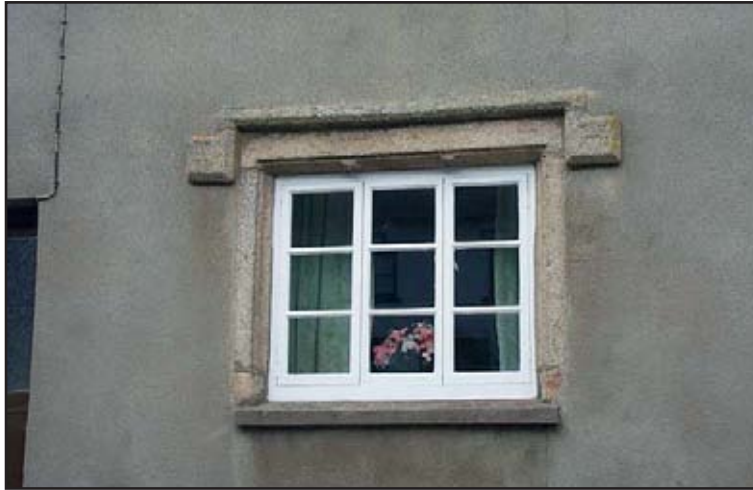
Fig 11 – Late 19th century style casement in late 16th century granite frame with hoodmould.
