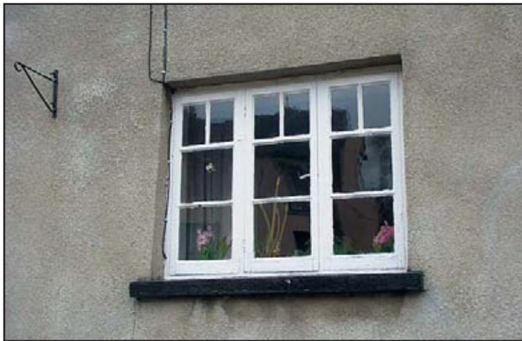
Fig 12 – One example of unusual casement subdivision.
