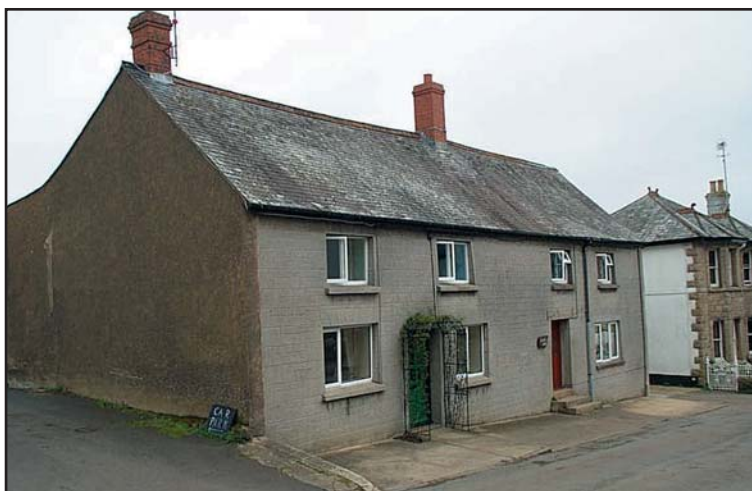
Fig 8 – Render imitating stone and coursed but roughly dressed stonework.
