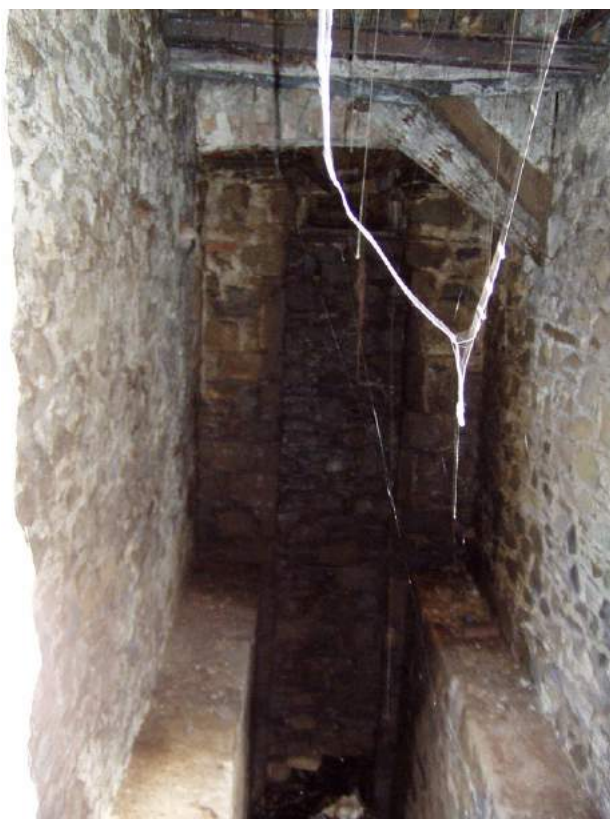
A rare example of a water-powered wheelpit in a bank barn. The wheel has been removed and no longer exists. © DNPA
