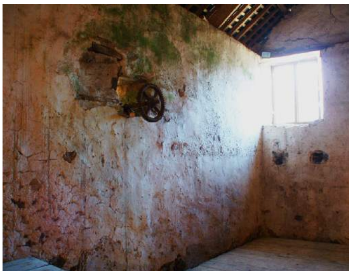
Gearwheel and usage marks indicating position of former fixed thresher. © Philip White
