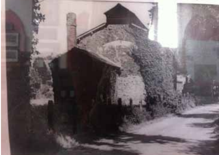
The back of the engine shed, as seen from Parish Road in 1947. The small annex, on the main building, was used as a stores/mess and equipped with cupboards and a table where the men could rest. For most of its existence the difference in floor levels result drop into the annex, but in the early 1930s the floor was raised with ash and clinker.
