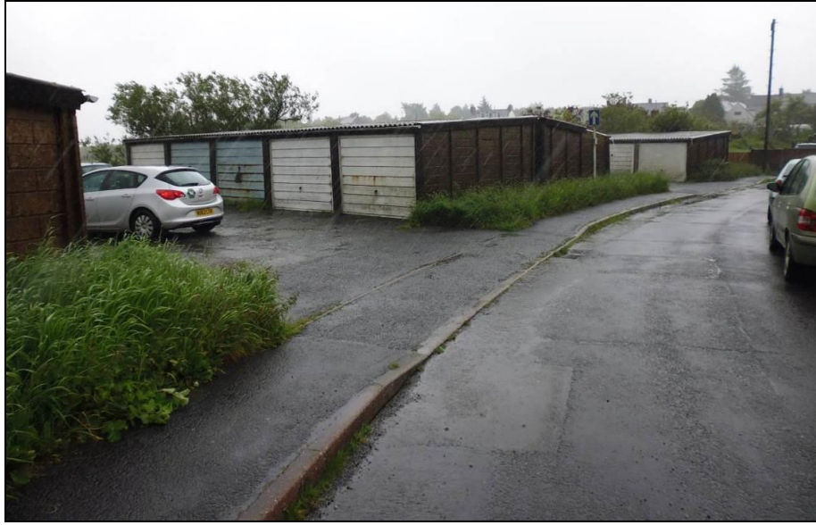
(Plot B: taken from the western boundary looking east)
