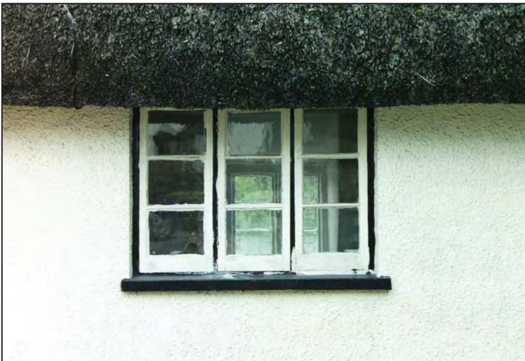
Figure 3 A typical flush-framed, multi-paned casement window
