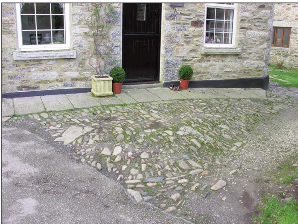
Figure 28 Rough cobbles, granite slabs and hoggin at The Cottage
