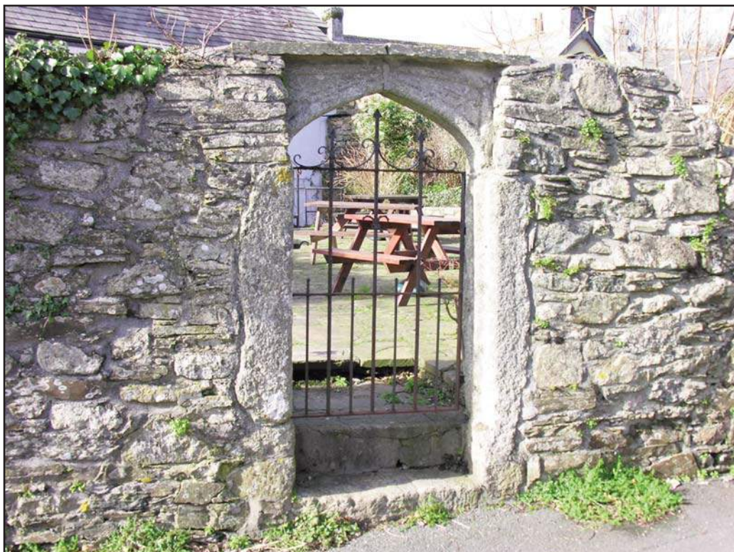
Figure 5 Granite doorframe
