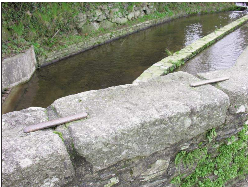
Figure 44 Coping stones to bridge parapet
