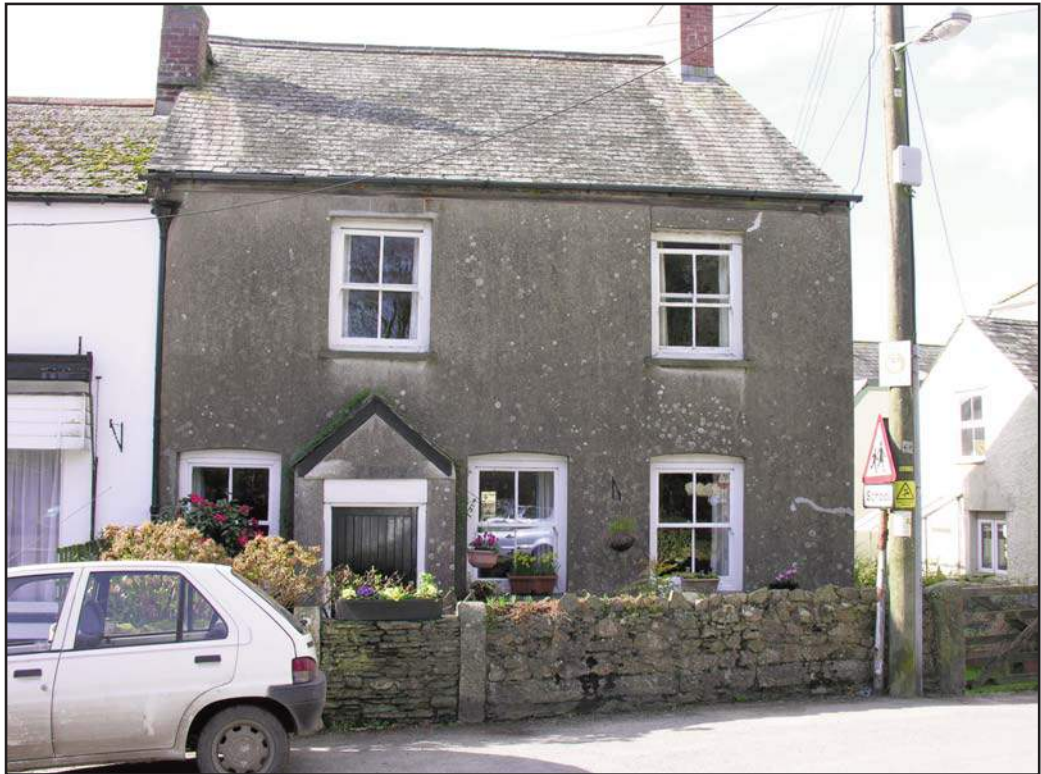
Figure 10 Brookside retains its original sash windows
