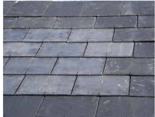
Solar slates incorporated on a natural slate roof
