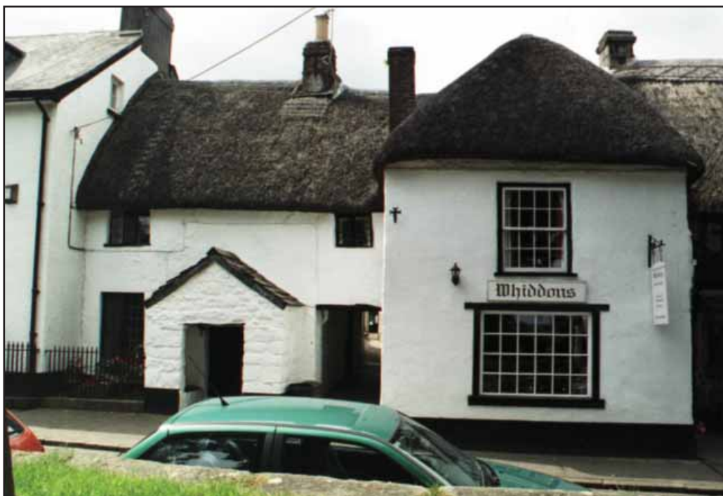
Figure 11 Whiddon's and Church Stile Cottage in High Street
