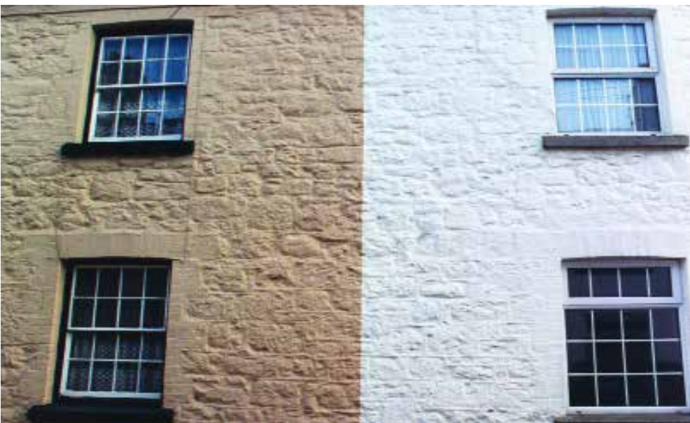
Figure 46 Traditional (left) and modern (right) windows
