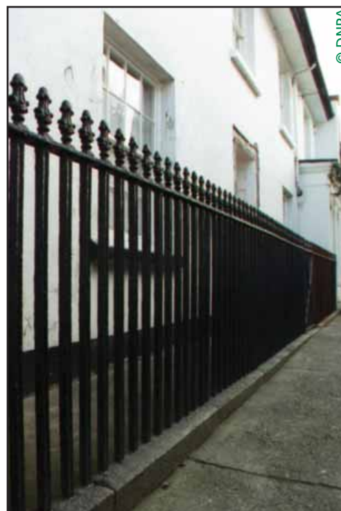
Figure 27 Railings in front of Dolphin House in Mill Street
