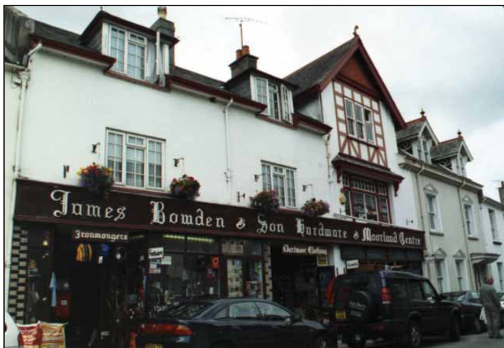
Figure 2 Early 20th century buildings on The Square
