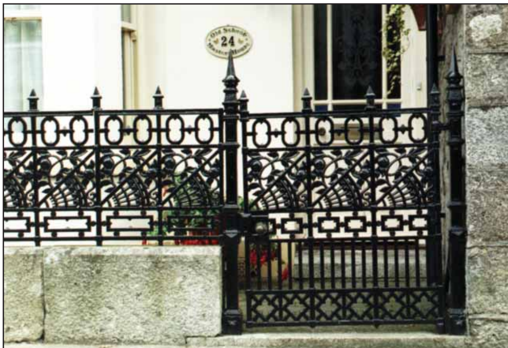
Figure 28 Gate and railings of the Old Schoolmaster's House, New Street
