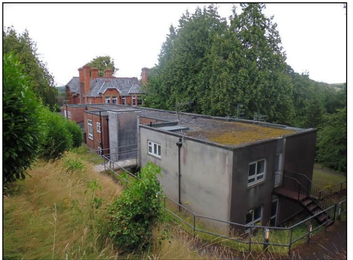
(View of the link and Kenwyn House from the western corner looking south east)
