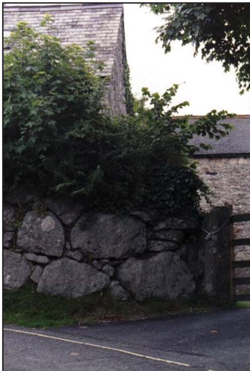
Figure 16 Large boulders used in wall construction
