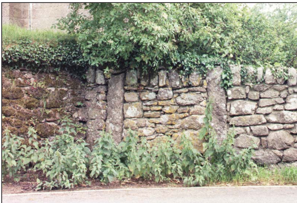
Figure 17 Evidence of former opening
