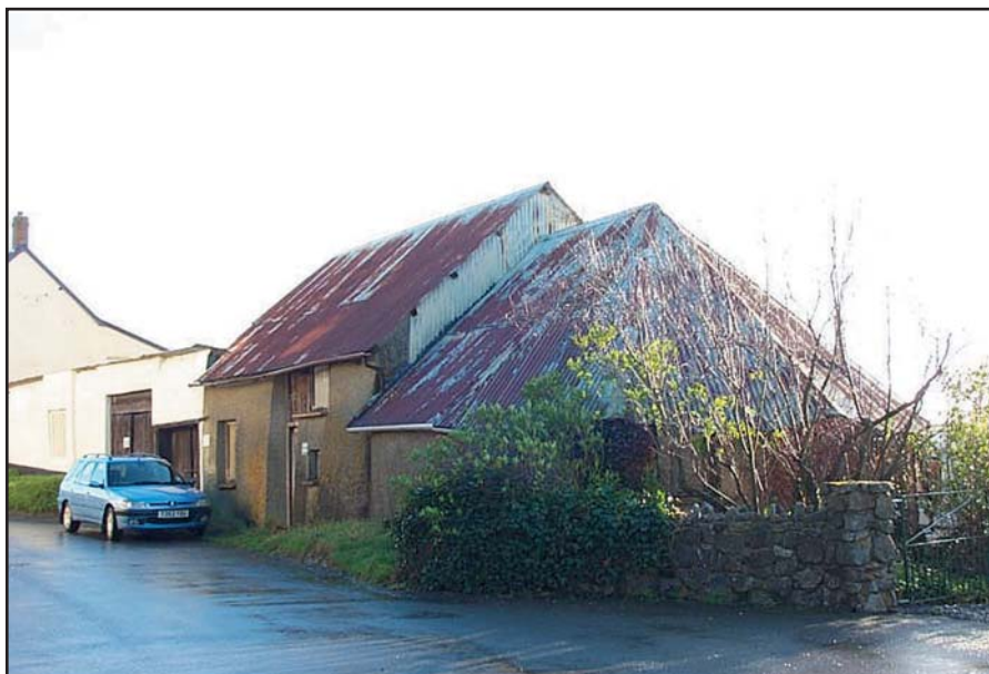
Fig 20: The thatch on this old barn was replaced with corrugated iron a long time ago
