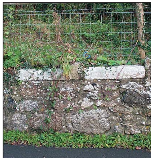
Fig 28: Rubble wall with granite slab coping near Doone Cottage
