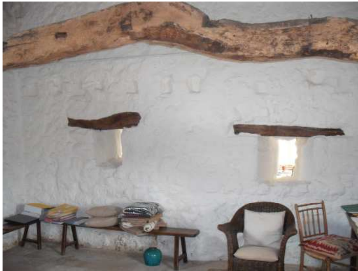
Figure 27. Remaining floor beam with joist sockets and corresponding sockets in the gable wall
