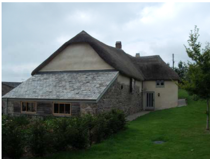
Figure 7. Middle Venton, approved shed/garden room reconstruction of a derelict outbuilding at the east gable end, beyond the lower end of the shippon, in the fore ground, approved rear extension in the background
