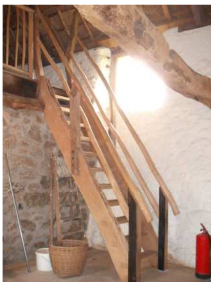
Figure 28. Steps and handrails
