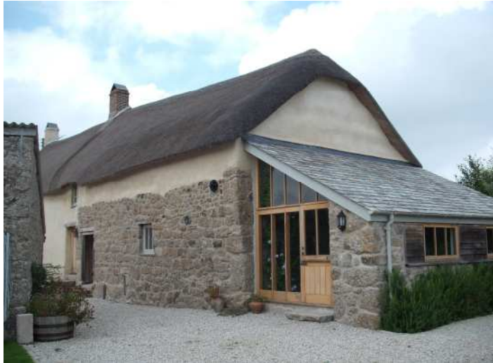
Figure 8. Shed/garden room extension created from derelict outbuilding abutting the shippon
