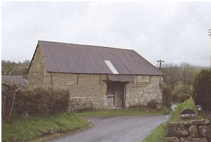
Figure 11. Threshing barn viewed from the lane, west elevation, listed grade II
