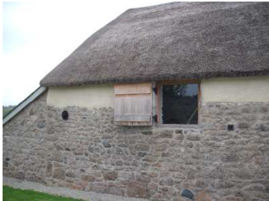
Figure 24. Glazing and shutter to the hayloft
