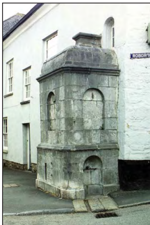
Figure 50 Conduit inset into house wall
