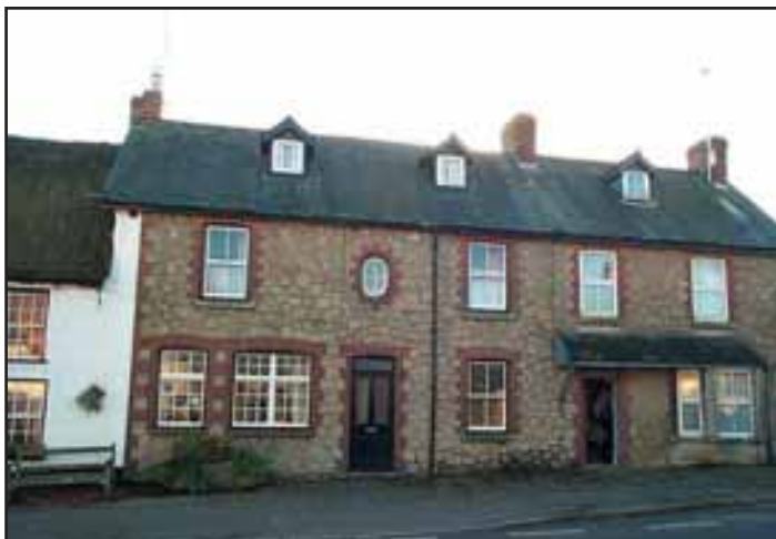
Fig 9 Victorian stone construction with a timber lean-to
