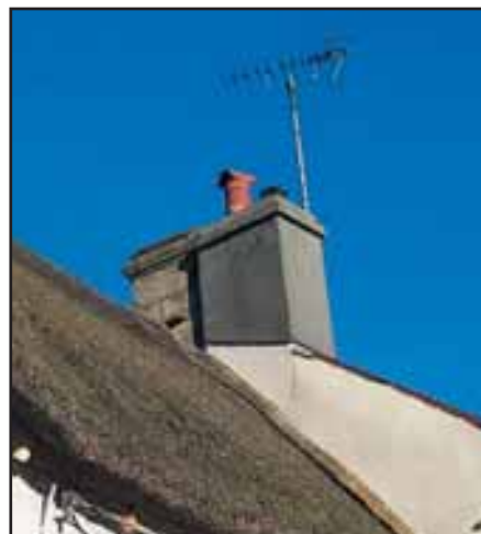
Fig 10 Dressed granite chimney at the Taw River Inn, partly obscured
