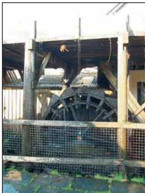
Fig 2 The elevated leat and one of the wheels at Finch Foundry
