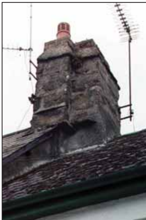
Figure 16 Early granite chimney stack with Weathering for thatched roof covering
