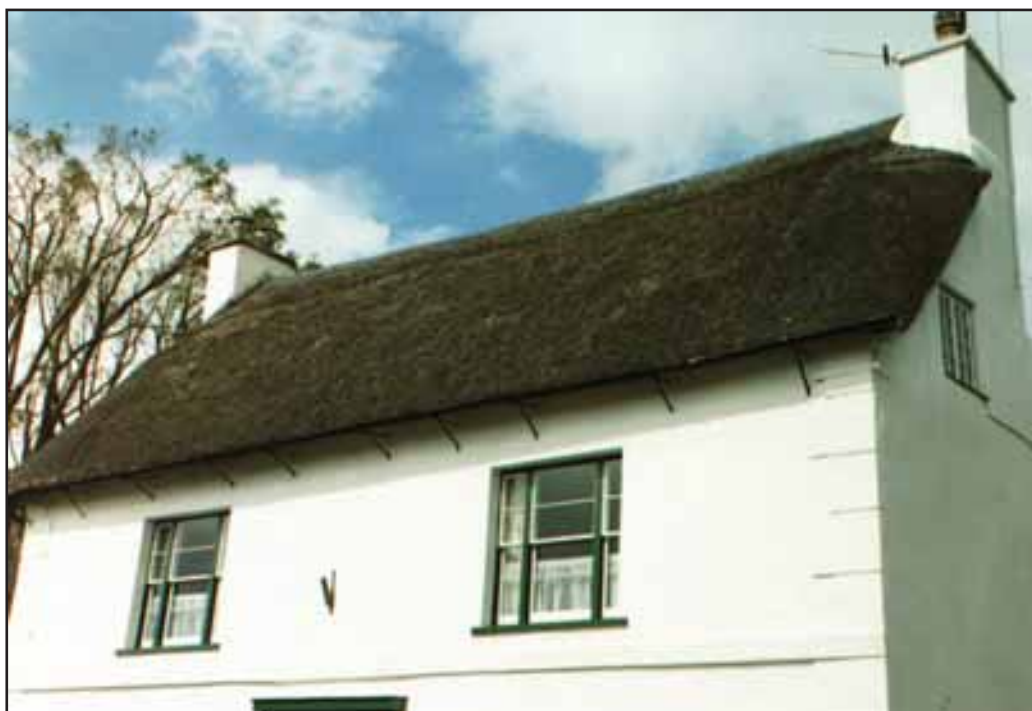
Figure 5 Thatched Roof of Greenhill House with flush ridge
