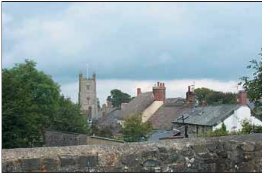
Figure 4 The attractive roofscape of Drewsteignton
