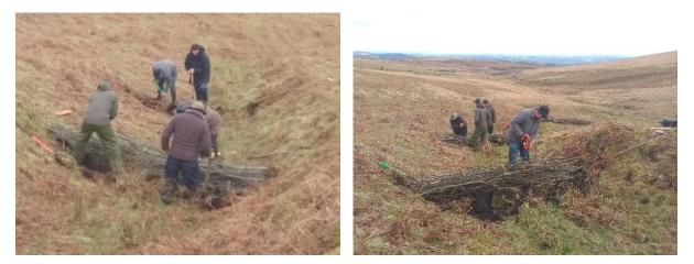
Leaky dams made from both live willow faggots and timber boards were installed into a network of old tin mining gullies, many of which channel significant flows during heavy rainfall.
