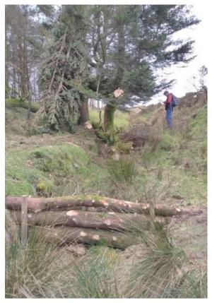
**Woody Debris dams** are made from fallen timber or material found locally on site and pegged securely in place. These dams blend in well with their surroundings, are naturally leaky and should remain in place for many years to come.
