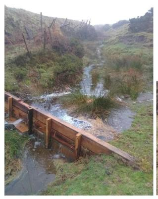
**Timber dams** on the left are holding back high flows from a network of tin mining gullies on Dean Common. They are made from untreated oak sleepers and will be resilient against weather and livestock interference. The lower boards have small spaces in between to allow leakage during normal flows.
