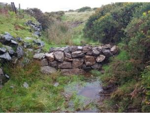
Water permeates slowly through the smaller stone on the downstream side of the structure, preventing erosion from any great force of water. These stone dams stood the test of storm Dennis, overtopping but without the loss of any stone.
