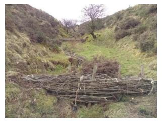
They are secured in channel with live willow stakes, which when growing will help to stabilise banks and eroded cuttings. The presence of the willow bundles in deeply cut, faster flowing channels will really help to break up and slow down the flow.
