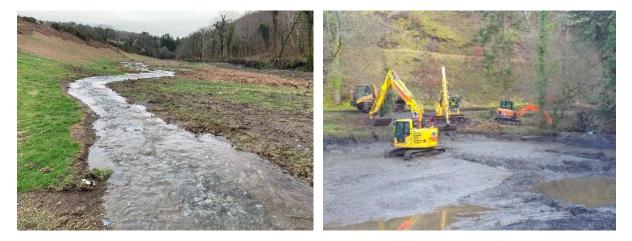
Finally downstream volumes of silt had built up in the sediment pond and lake due to the speed and volume of water heading downstream. Both pond and lake were cleared of silt and the measures put in place should reduce the silt load in future, allowing more water to be stored in the lake. This project will be closely monitored over the coming years to measure the effects on flow, silt deposition and biodiversity.
