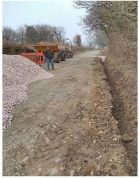
Houses in Scorriton have been flooded very recently as a result of flood water running down the driftway into the village. In a joint project between the Ranger Service and the Headwaters Project drainage improvements have been carried out, to include new French drains, renewed cross drains and a series of trial infiltration pits to soak away the water.
