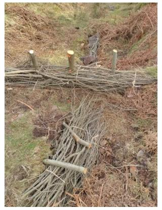
of the gully and are also pegged down lengthways into deeply eroded channels and erosion holes to prevent further damage.
