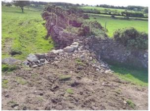
Normal flows pass through the leaky dams unimpeded; it is peak flows that are slowed and stored to ease the pressure downstream.
