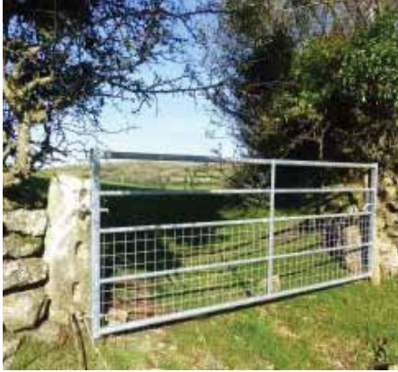
Original five-hole gateposts converted to make a modern gateway
